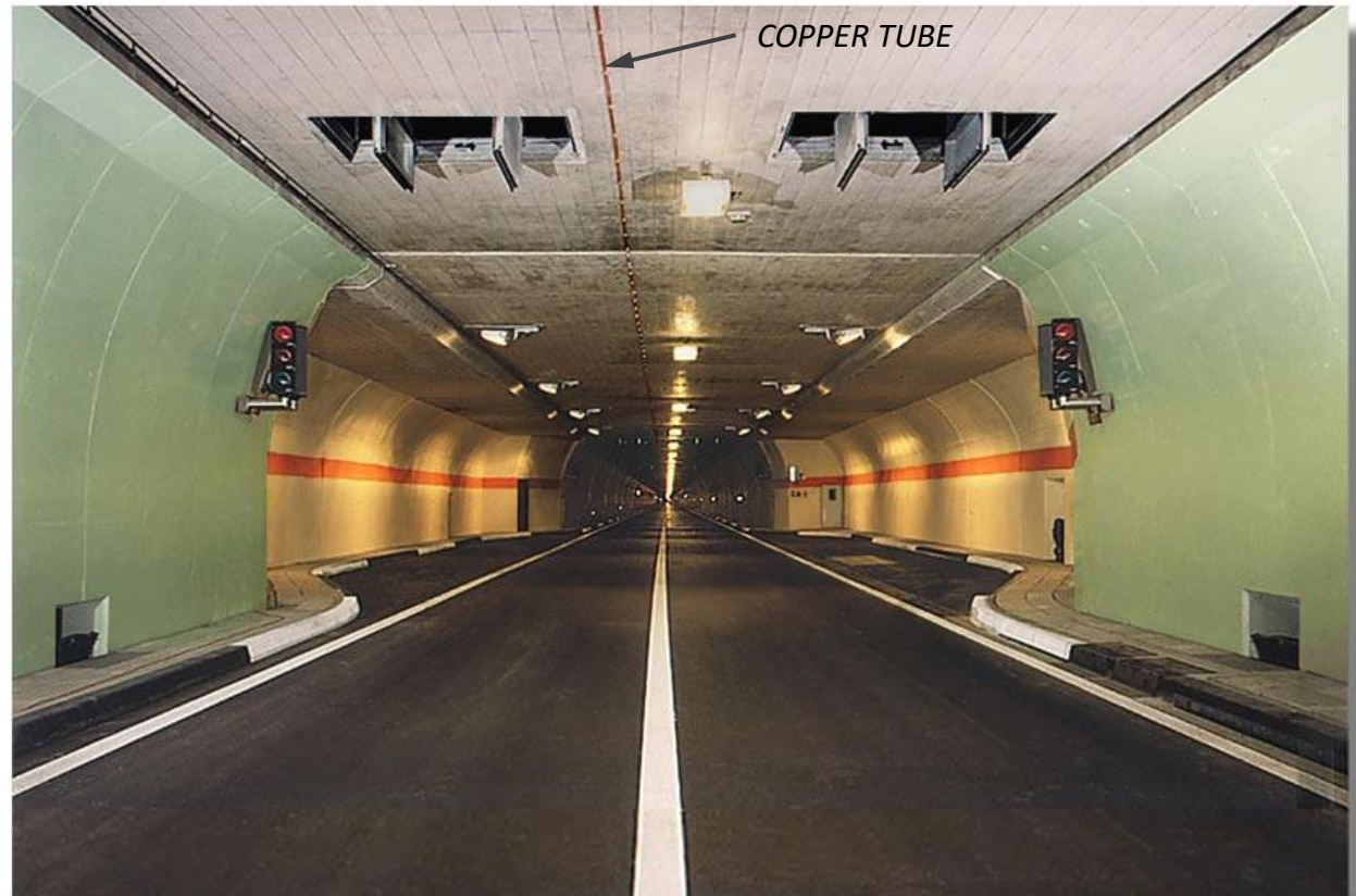
2.5km Bypass Tunnel
